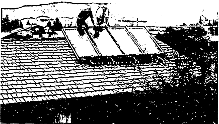
In the energy conscious era of the 1970s, NASA's operational experience found many new applications. This prototype water heater, warmed by solar cells, was installed on a home in Idaho.
